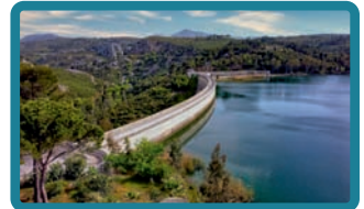
Use Case #3: Synchronized attack on water treatment facilities
